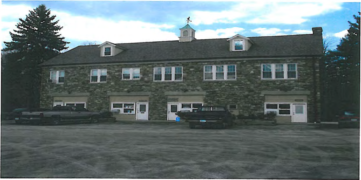
Photo above is the rear view of the Beekman Town Hall, see the lower level, which depicts four large tan and white wooden window and access door areas which are actually infills for what was once the four overhead door openings where the fire, rescue and highway equipment was stored. Source : EMAPS Assoc. March 2006.
