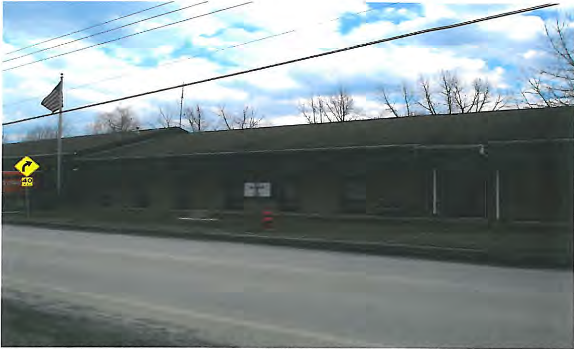
The Photo above is the front view of the Beekman Fire House, which extends westerly beyond the apparatus bays, view from CR7. Source : EMAPS Assoc. March 2006.
